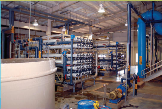
Water/Wastewater Treatment Plants
